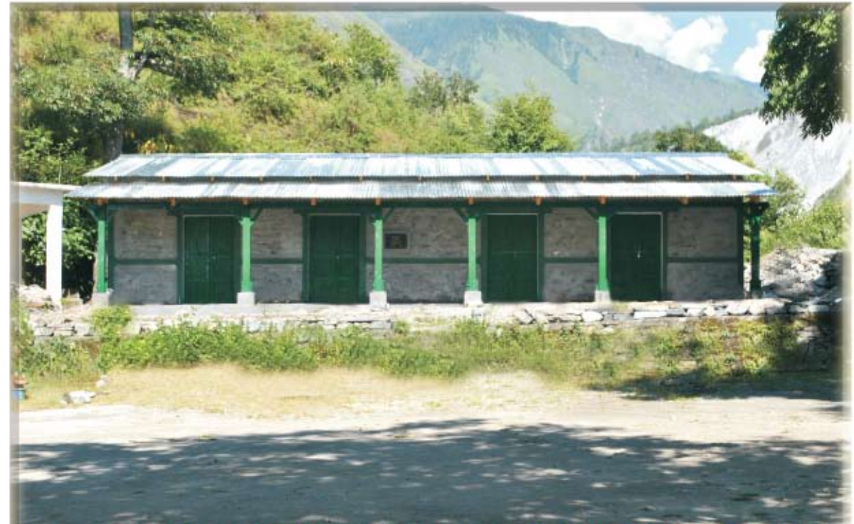
Inauguration of Two School buildings at Gauna, Chamoli District
